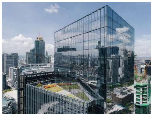
ARTHALAND Century Pacific Tower (ACPT), a mixed-used commercial building located in Taguig business district, is the first in the world to receive EDGE Zero Carbon Certification. The tower has offset 100 percent of its operational emissions and with projected energy savings of 45.0 percent (Source: EDGE Buildings Facebook page)
