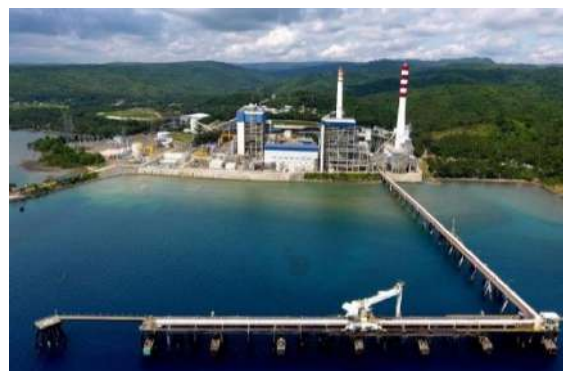
The 500-MW supercritical coal-fired power plant of San Buenaventura Power Ltd. Co. in Mauban, Quezon (source: tribune.net.ph)
