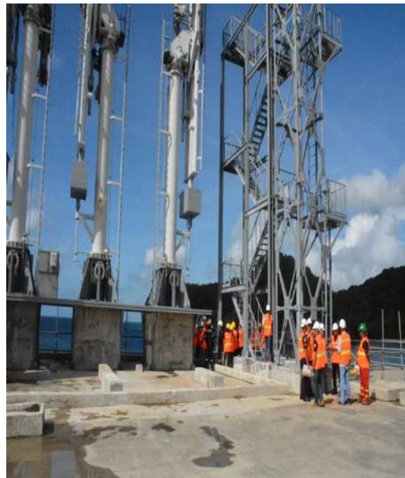
Regular Inspection & Monitoring of Natural Gas Facilities in the Philippines
